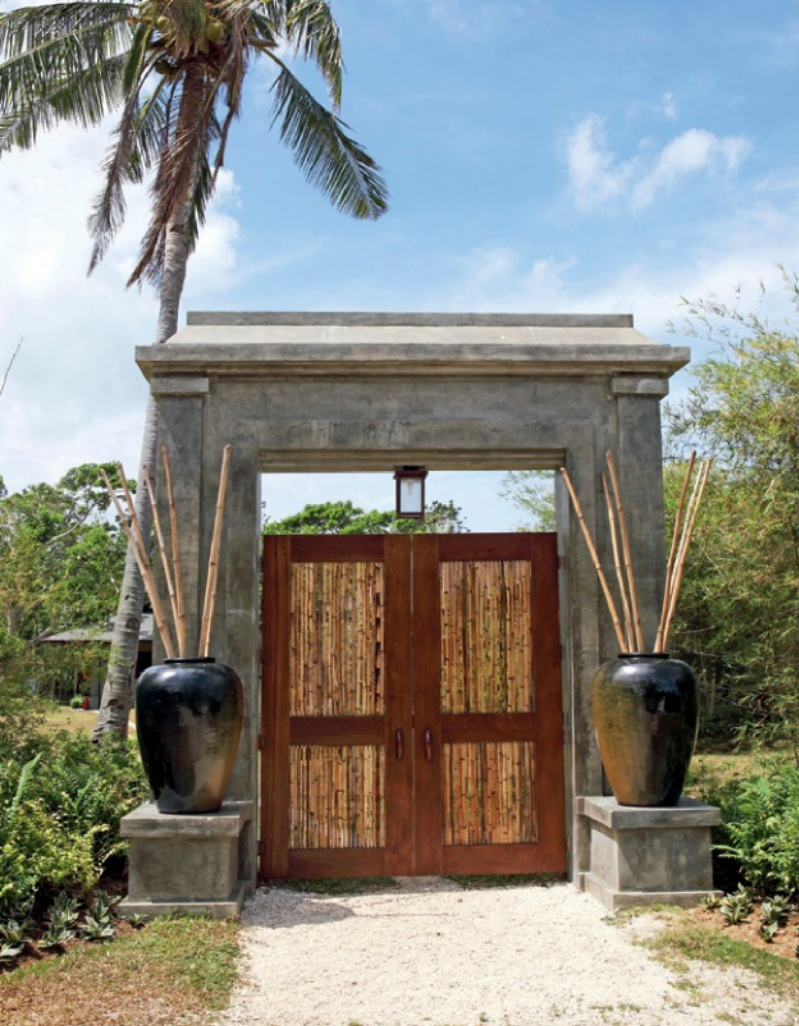
The main portal into the estate is finished in runo . An imposing concrete structure frames it while overscaled planters on concrete pedestals frame it.
